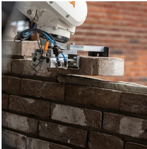
Figure 13 The Ropax robot for bricklaying (Source: Ballast Nedam)
